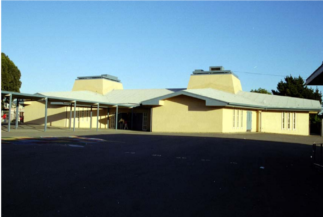
Figure 12: Front of Pod Classroom Building
