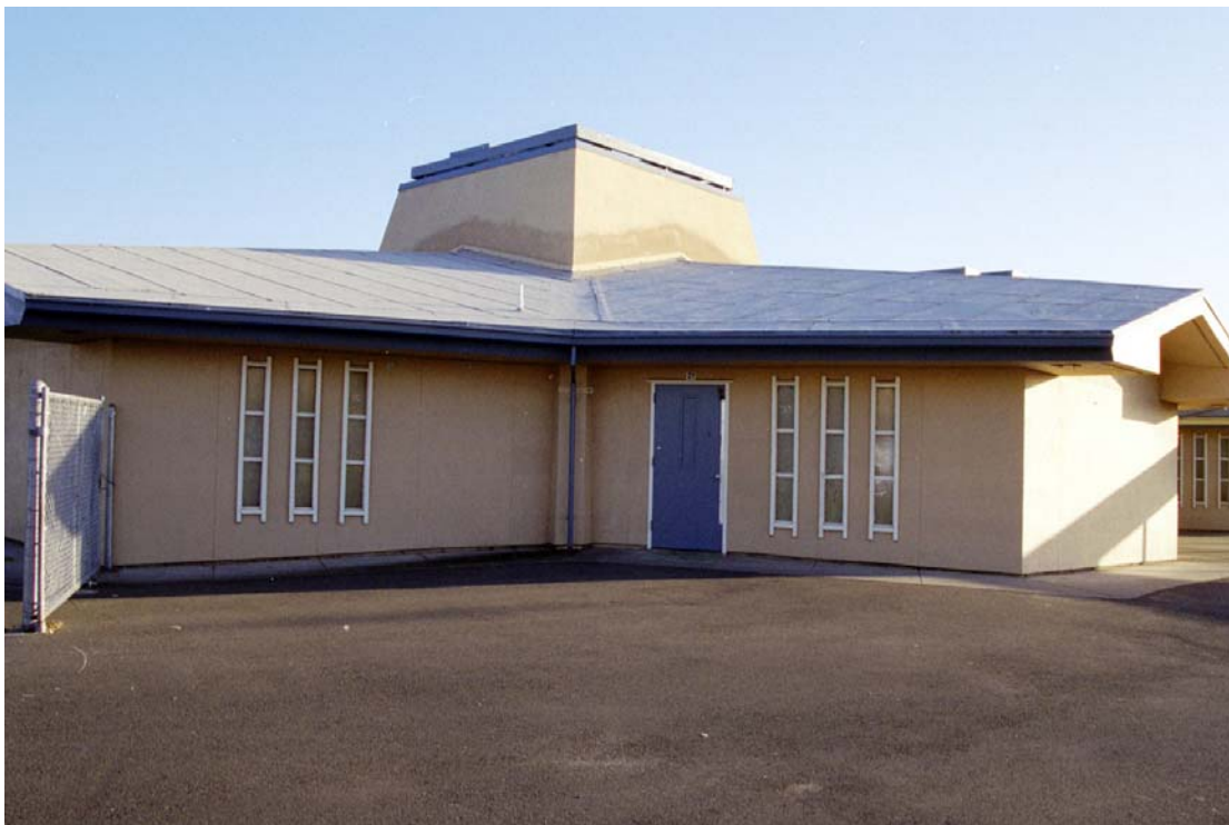
Figure 13: Pod Classroom Building
