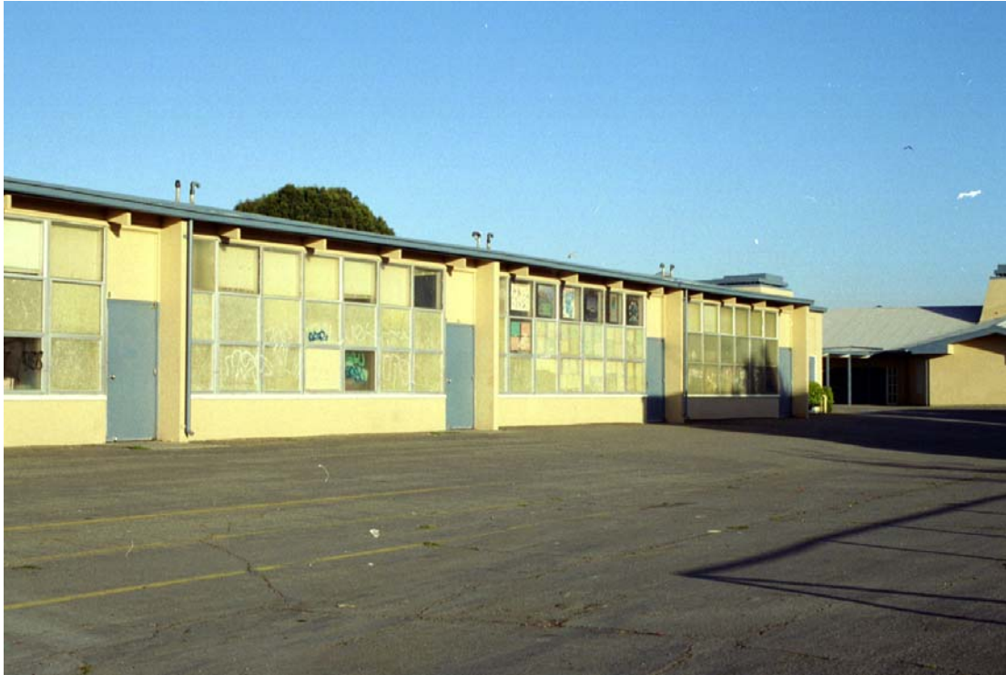
Figure 8: South Side Classroom Bldg.
