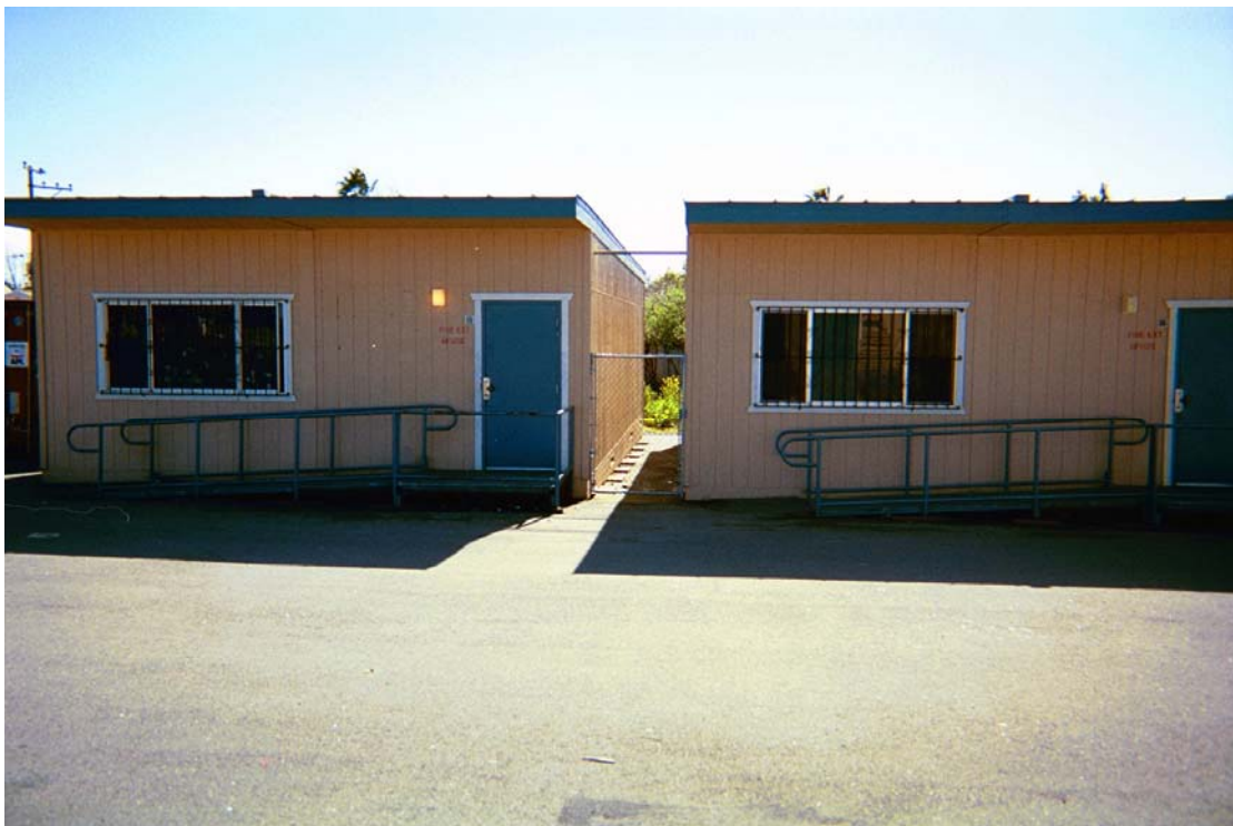
Figure 15: Portable Classroom Building Connected with Electrical Conduit.
