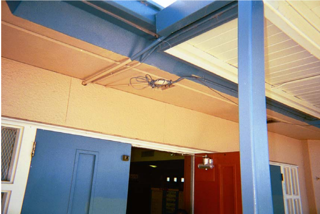
Figure 14: Conduit Crossing Seismic Joint at Unit A
