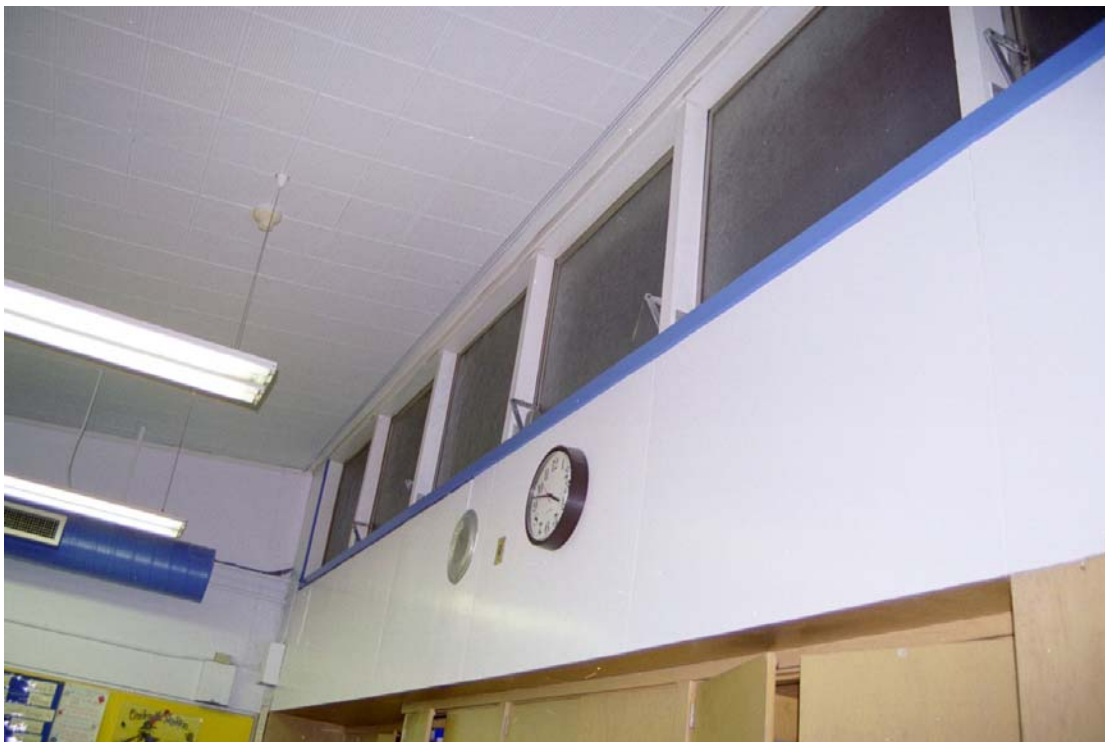
Figure 7: Clerestory Windows at Classroom.
