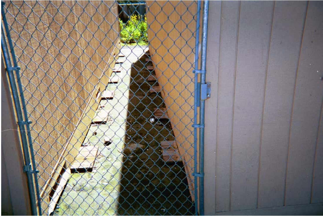
Figure 16: Portable Buildings Resting on Ground.
